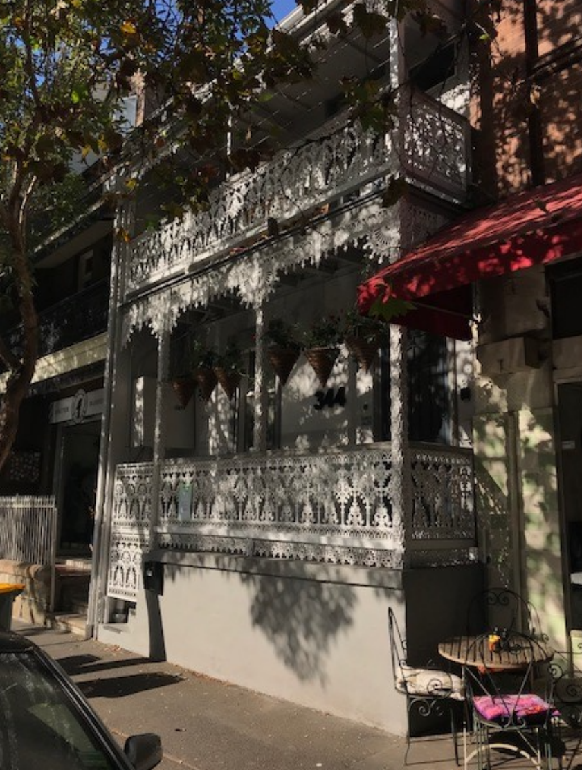
Figure 2: Site viewed from Crown Street
