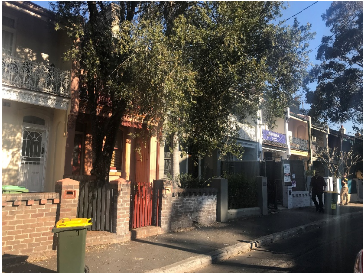
Figure 3: Looking west along Charles Street
