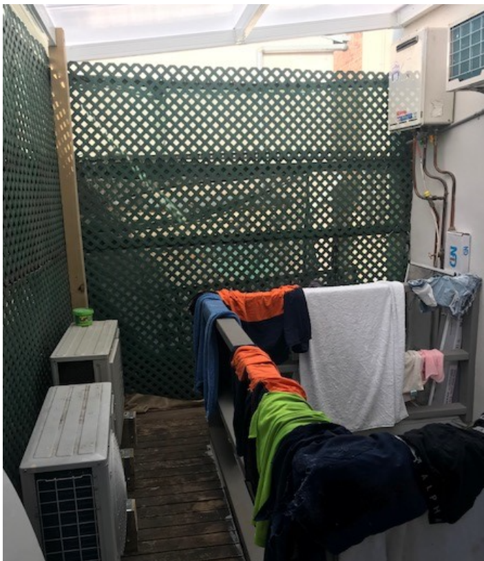
Figure 4: The second floor courtyard
